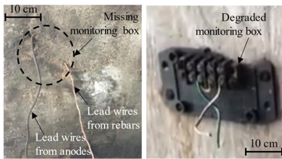
(a) Missing, naturally degraded/damaged monitoring boxes
