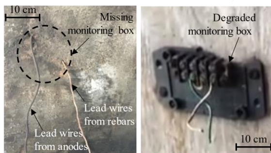
(a) Missing, naturally degraded/damaged monitoring boxes
