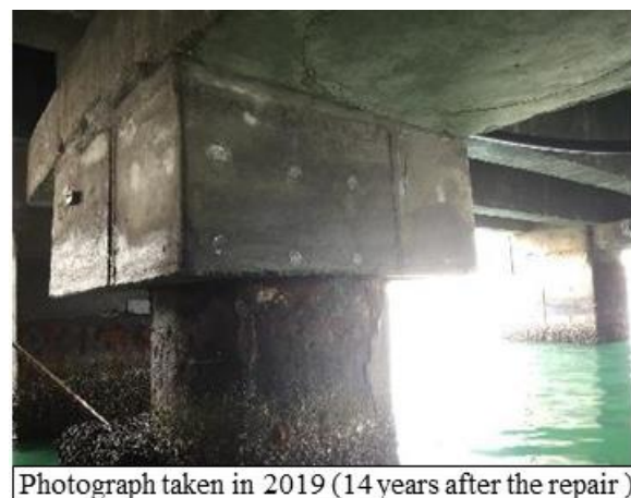
(b) CP protected pier after 14 years
